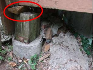
Observation #4.4: The exterior stone and wood stairs were significantly deteriorated and not stable.
