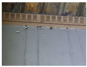
Observation #4.6: In multiple locations, the stone siding in front of the foundation wall cracked/loose/missing and exposing the waterproofing/insulation/foundation behind. Some of the insulation was also observed to be missing.
