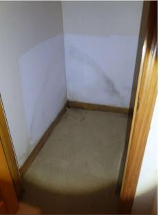
Observation #10.4: The bottom of the masonry wall in the garage space appeared to have black mold stains.
