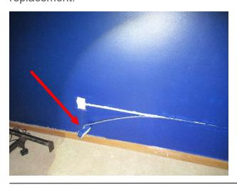
Observation #7.12: Multiple receptacle outlets were malfunction and missing cover plate Implication: Possible safety hazard
