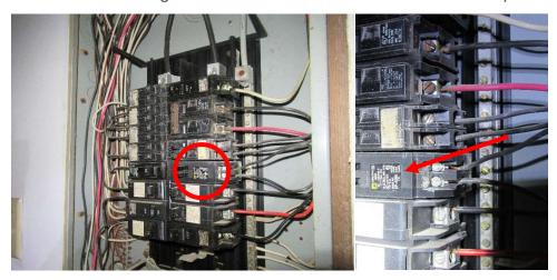
Observation #7.8: Visible corrosion on the screw inside electrical panels Implication: Indicate excessive moisture condition in the basement area Comment: Recommends hiring an electrician for further evaluation, repair and replacement.
