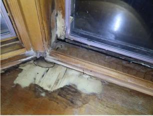
Observation #10.7: The hardwood floor finish in a closet on the 1<sup>st</sup> floor appeared to have water damaged and is loose.
