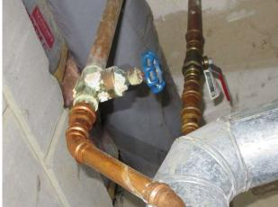
Observation #6.14: Visible water leaks in the drainage piping system in the basement Implication: Possible water damage to interior home space
