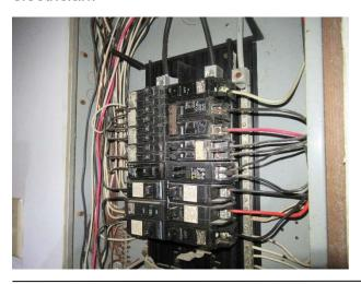
Observation #7.10: The neutral bus bar and ground bus bas was connected in the subpanel.
