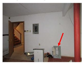
Observation #7.6: Tandem circuit breakers were installed in the electrical panel which was not allow per panelboard diagram.
