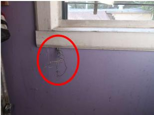
Observation #8.5: Live electrical wires hanging on the basement ceiling near the electrical panels
