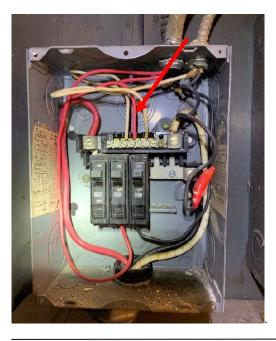
Observation #8.7: Most of the breakers installed do not match the electrical panel brand.
