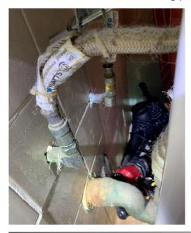
Observation #7.4: The cast iron wastewater cleanout cap was missing.
